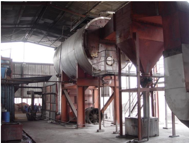
EFB fired steam boiler at 450 kWe CHP plant of Juaben oil mill, Ghana
