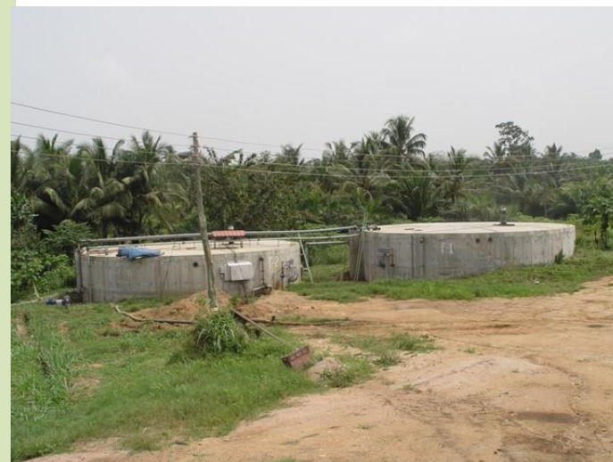
900m 3 biogas system running on fruit processing wastes at HPW Fresh& Dry in Ghana
