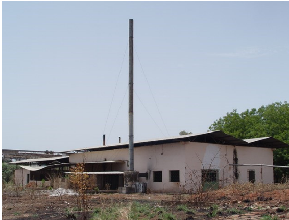
Figure 23: SICAJU power plant
