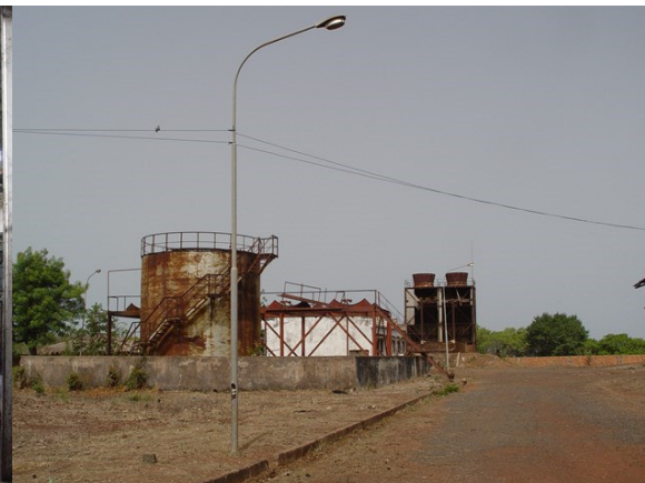
Figure 36: Bafata power plant premises
