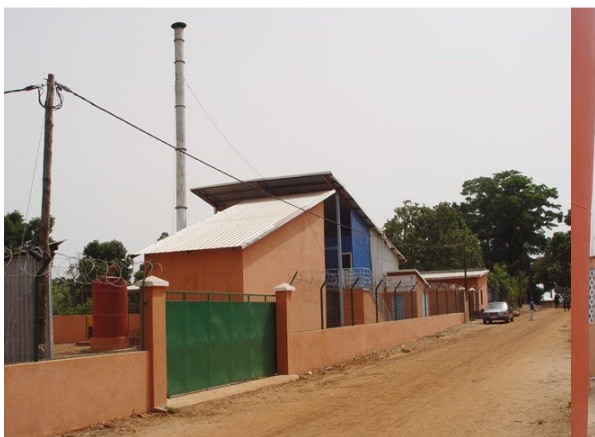
Figure 19: SAFIM power plant
