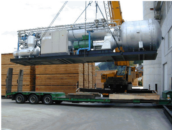
Figure 1: 400 kWe ORC unit in Admont (Austria)
