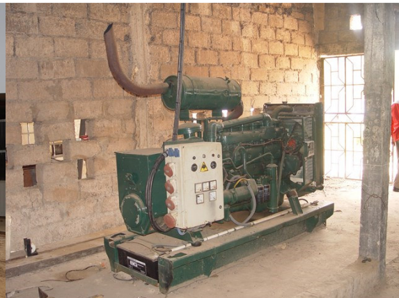
Figure 37: ARREY cashew processing plant in Bula Figure 38: 100 kVA diesel generator at ARREY
