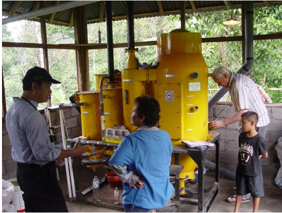
Figure 3: 25 kW rice husk gasifier in Indonesia
